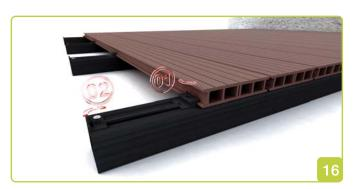
To fix the final plank, simply screw the end clip into position using the previous centre clip as a locator (Fig 16). Repeat the action of engaging the plank in the centre clip, then push the board into position, making sure that the end clip locks the final plank in place as you did for the first plank (Fig 9).
