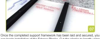
can begin installation of the Edenex Planks. Cut the planks to length using a power saw with fine tooth carbide blade allowing for the expansion gaps mentioned above. Make allowance for expansion in length of 3mm per metre length on all planks and 3mm in width in each plank
