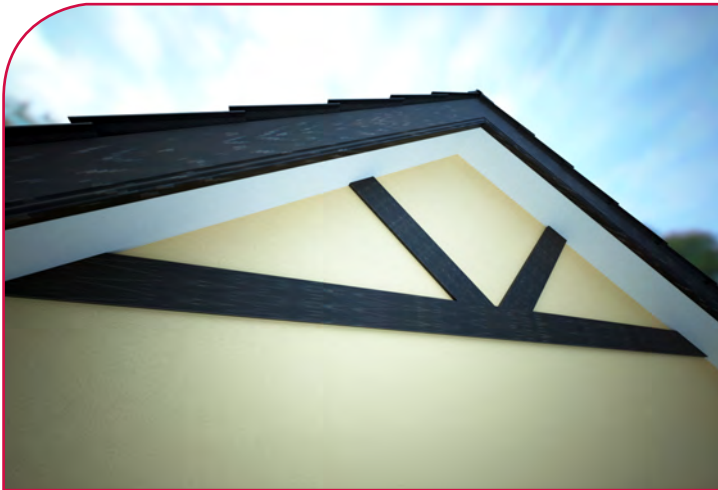
1. Tudor board installation
