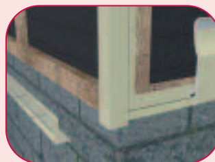
fig 8 Showing starter trim and showing the use of the universal corner trim for external angles
