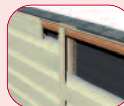
fig 11 Top edge detail showing packing piece and 2-part Universal trim.
