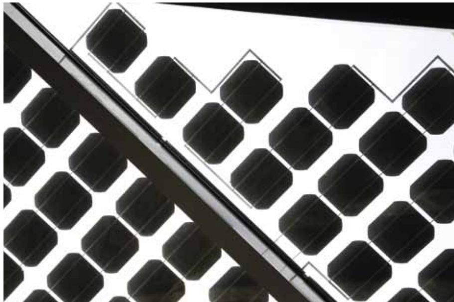
In order to maximise the output of the 45° angle curtain wall, special glass-modules were made with custom connected cells that fit the hospital's eye-shaped public hall.
