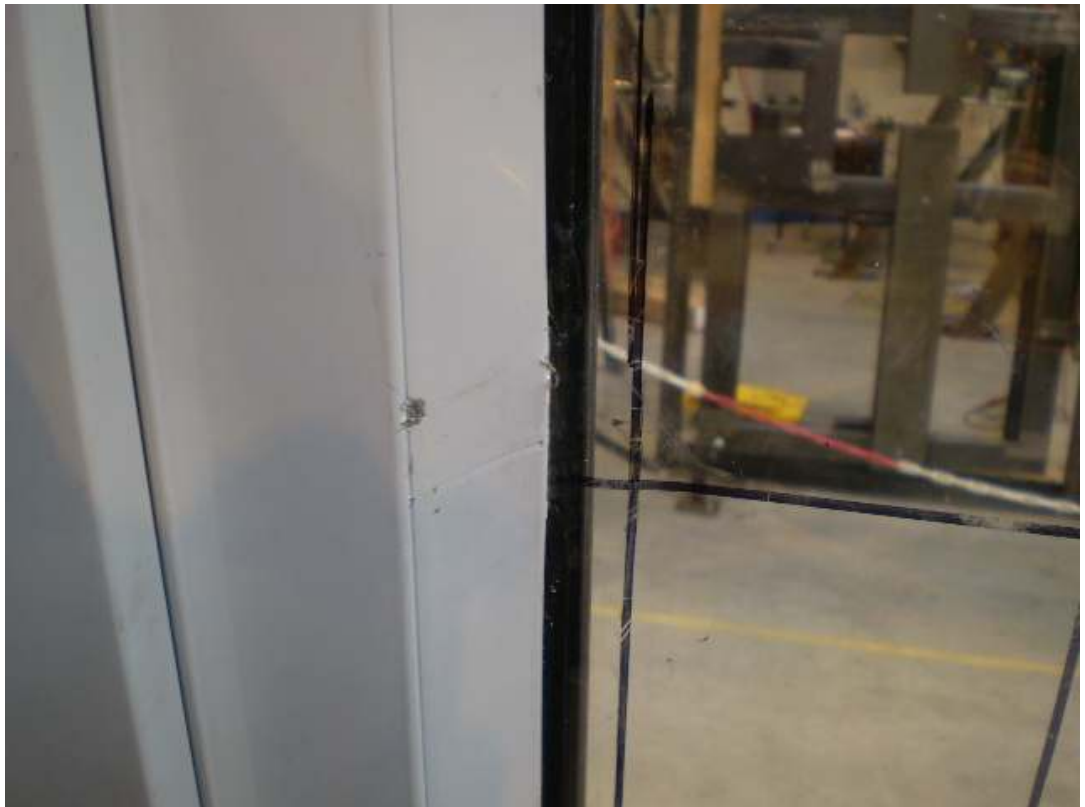
Damage to the glazing gasket following basic security test
